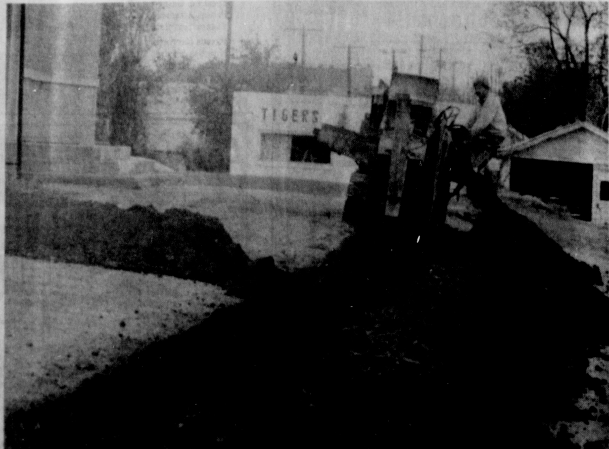
REPLACING THE DAMAGED pipes at McLean High School has made a big mess of the school grounds as workers have had to dig a series of trenches to lay new pipe. The plumbing was damaged in a recent thunder storm when a lightning bolt hit the school. (Photo by Linda Haynes)
