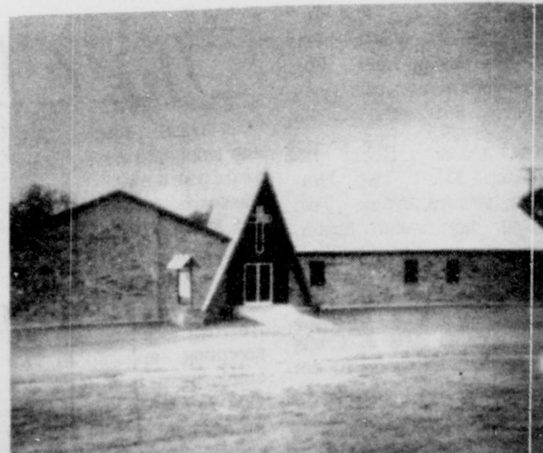
Assembly of God Church was chosen "Most Improved Facility" of the month. Taking two years from start to finish, the building now has new windows and a new brick exterior.
