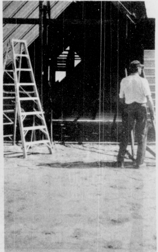
When the Cross is raised, workers will have to wait for an extremely calm day or perhaps do it at night. Pictured above is the center section of the 190 foot Cross. The picture left is a shot of the inside of the structure. Platforms and ladders fill the interior space. If a worker was to fall while working on the interior, they would not fall more than 8 to 10 feet.
