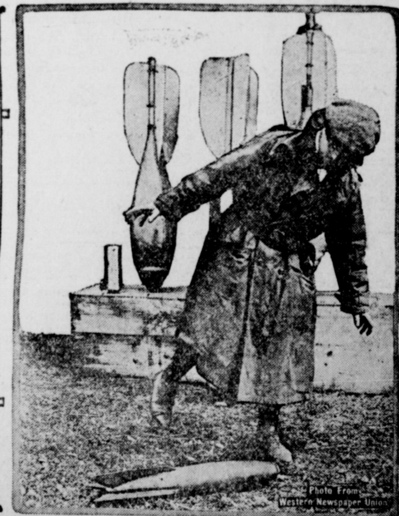
Several types of airplane bombs invented by Americans and adopted by the United States government are shown in the illustration. The man is kicking one of the missiles to show that it is harmless unless its nose hits something.
