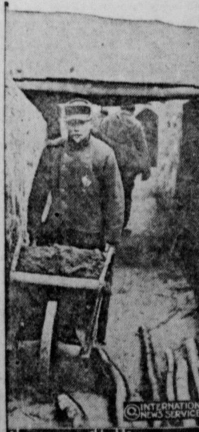
One of the deep trenches on the firing line in northern France. The allies have constructed hundreds of miles of ditches like this.
