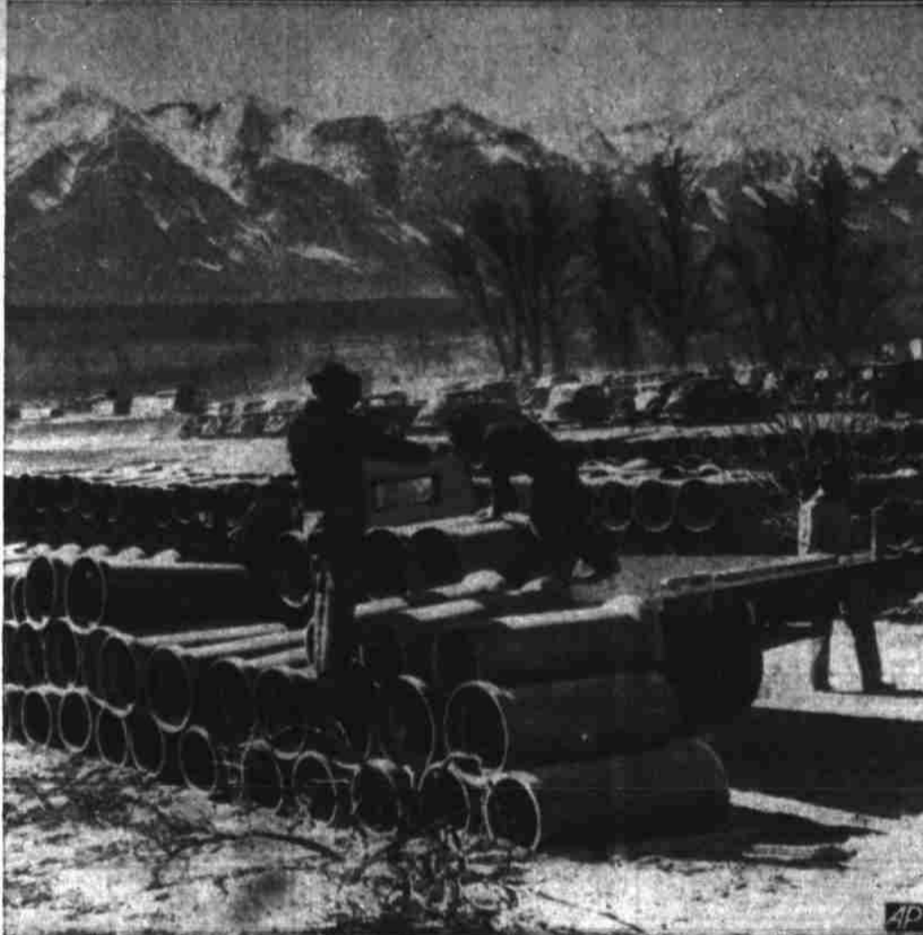
PIPES NOT OF PEACE —At Manzanar in the Owens river valley area of California, pipes for use in construction of a camp for the housing of Japanese aliens arrive. Manzanar is about 235 miles northeast of Los Angeles and near Sequoia national park. Already 1,000 Japs have headed for the camp, which eventually will house 10,000 persons under U.S. guard.
