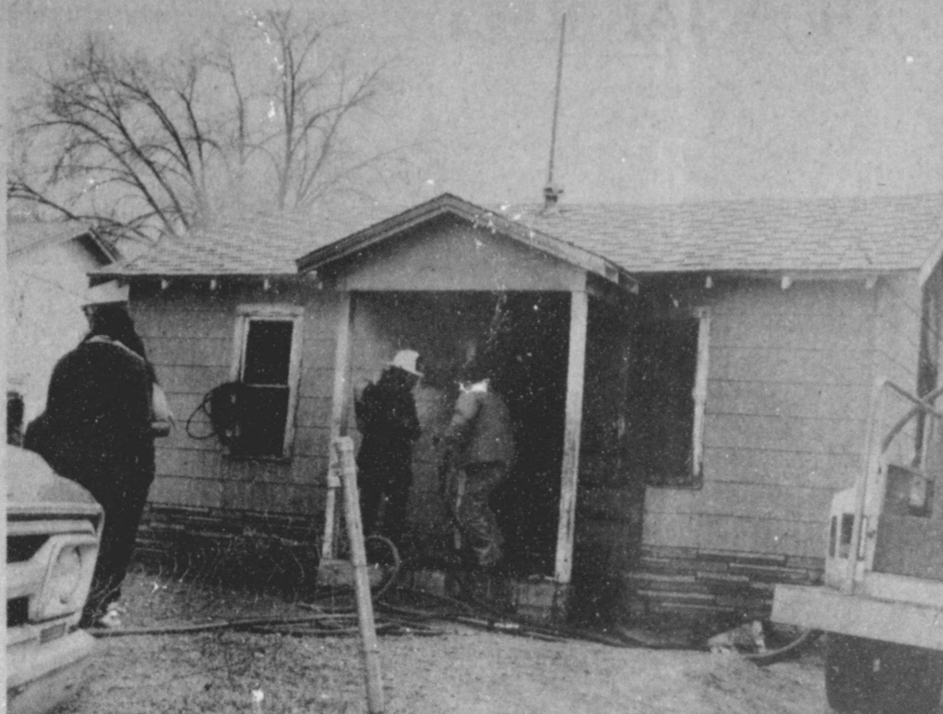
FIRE DAMAGES HOME --The Lupe Gloria home on East Fourth Street in Muleshoe was the first fire loss of the year. The home received heavy damage to the living room and lesser damage to the kitchen in a blaze on New Year's Day. Fire officials have not determined the cause of the fire.
