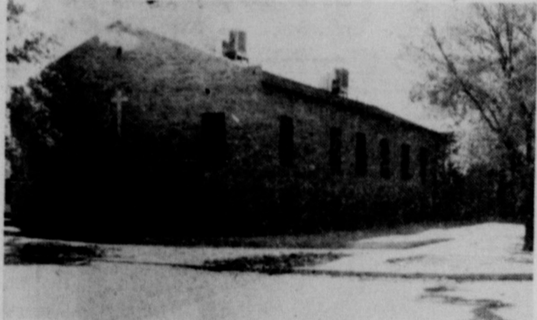
Only this year was work completed on the complete remodeling of the sanctuary of the light brick building. This is a picture of the north side of the sanctuary, entrance to which is made either on the northwest end or the southwest end. The pulpit, formerly located in the west end, is now in the east end of the sanctuary. (Photo by Payne).
