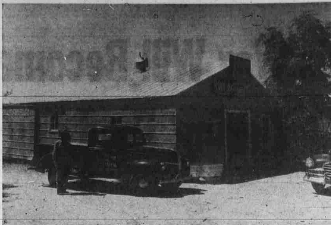
Roofing Company —One of the major firms of its type in West Texas is the Underwood Roofing company, located at 302 Lancaster and pictured here. It is owned and operated by J. E. Underwood who has established an outstanding reputation in roof construction and repair, during the nine years of operation here. With limitations of wartime on construction materials, Underwood stresses the importance of keeping roofs in good repair, so that whole structures are properly protected. (Kelsey Photo).
