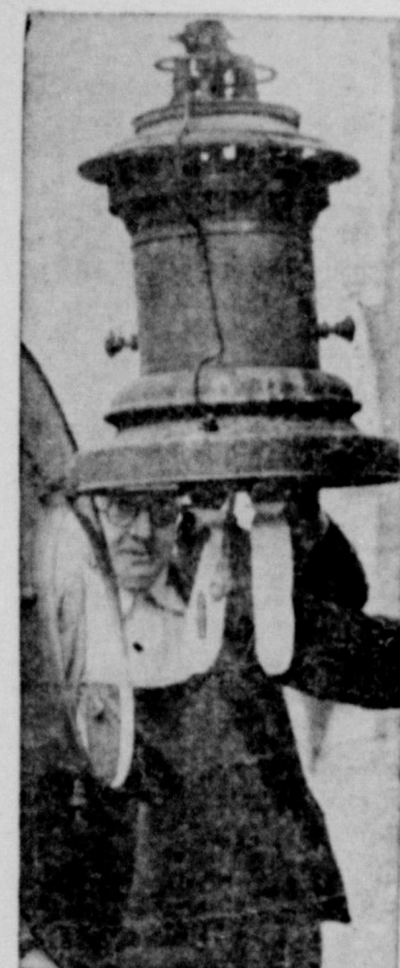
NEARLY AS WEIRD —Outlandish device being held by this workman is one of London's gas lamps. Extra hand in the picture belongs to the chap who is replacing a mantle, meanwhile holding the lamp's globe on his head.
