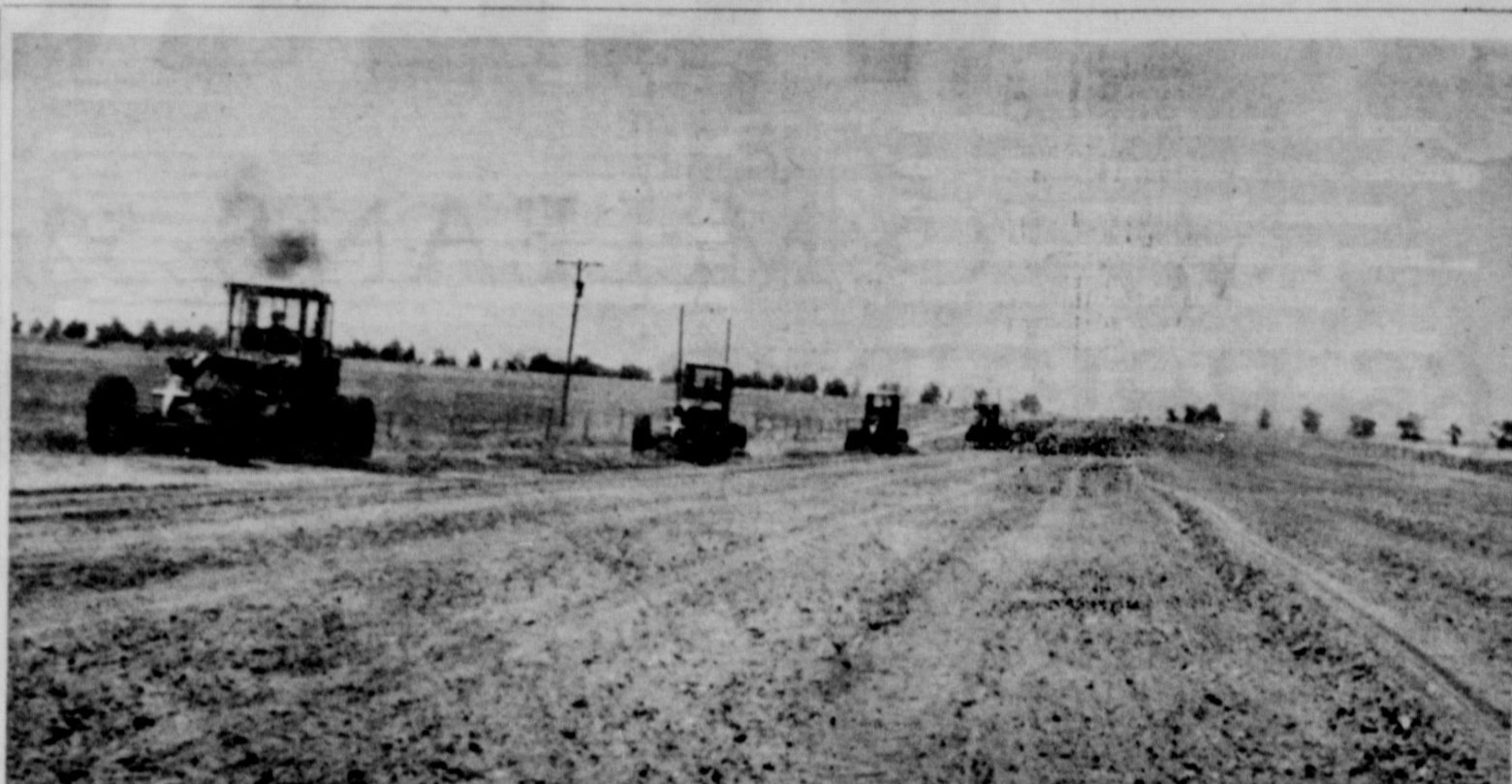
HARD AT WORK: Four Gray County graders swing into action on the McLean Municipal Airport runway project, northeast of town. The landing strip, previously inadequate for serving any but small aircraft, is being leveled, smoothed and oiled to provide a better landing service in a joint project of the county and the City of McLean. County Commissioner Truitt Johnson reported this week that 15,000 gallons of oil had been poured on the runway, and a smooth, hard surface is expected to result. (McLean News Photo)
