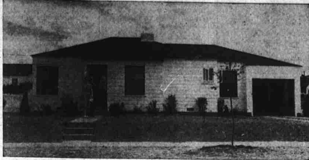
"Texan" Home —Pictured above is the "Texan" demonstration home, being shown to the public here this week in observance of Texas Home Building Week. Through the house was constructed by Wm. Cameron and company, with Taylor Electric and Runyan Plumbing company cooperating, and with Barrow's furnishing the unit for display purposes. It's an example of what may be constructed at less-than-rental payments. (Kelsey Photo).
