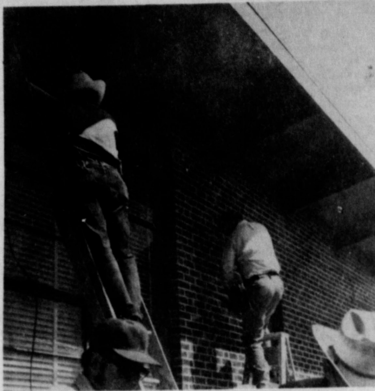
VOLUNTEERS INSTALL AIR CONDITIONERS
