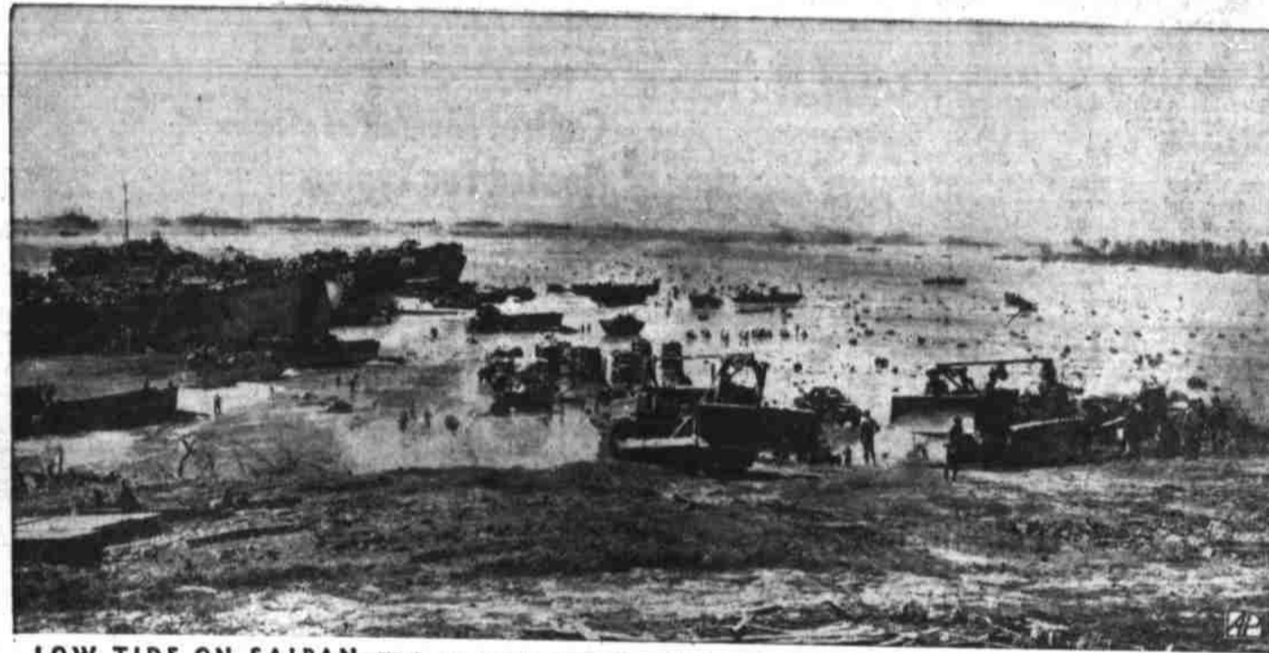
LOW TIDE ON SAIPAN —While vessels of a convoy lie on the hazy horizon, bulldozers on the Saipan beach pull trucks up a new roadway at low tide. Several LCM's have been caught on coral flats by the receding water.
