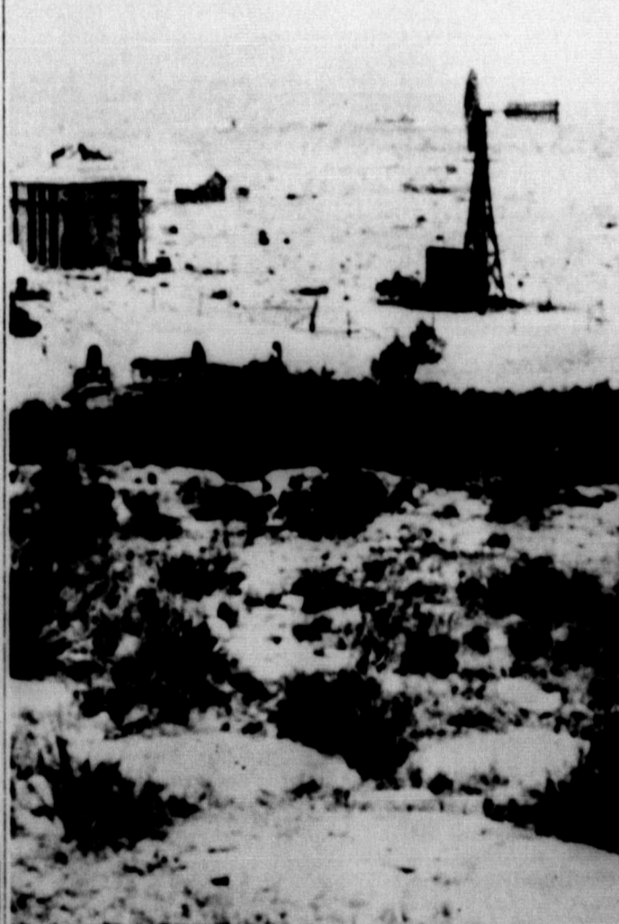
FIRST WATER WELL in all the vast reaches of Crockett County was located in the heart of early-day Ozona. The windmill on its wooden tower and the cypress tank and trough provided water for the entire population, for domestic and livestock watering. Note the dirt road leading in from the west, upper center, winding its way directly to the windmill. The big tree to the right center of the picture is the then youthful liveoak tree under which the first Crockett County Commissioners Court held its first meeting after the county's organization in 1891. The big tree, now much larger, is in front of the Baptist Parsonage and is marked with a bronze plaque. The First Baptist Church is built directly over
