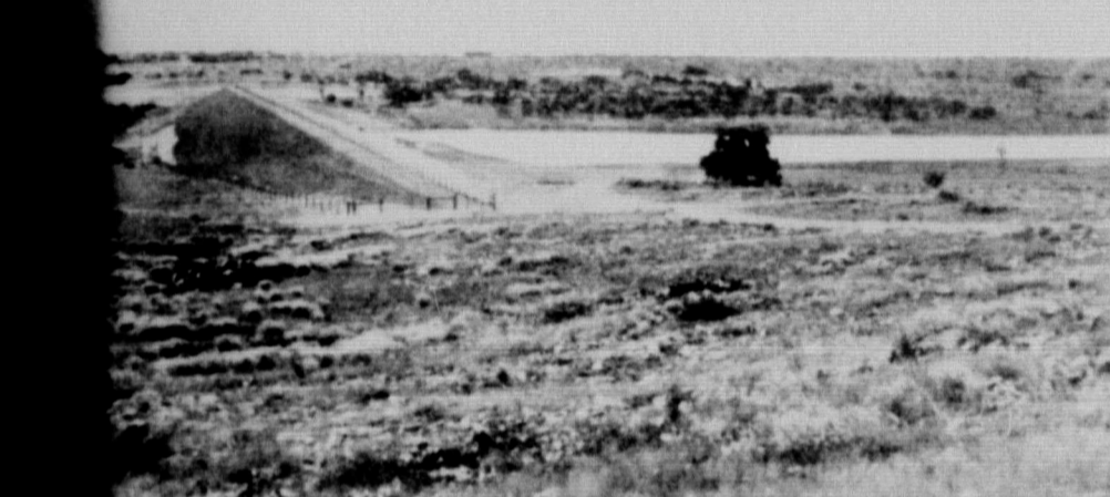
CONTROL DAM at work. The small lake of water is being held up by this flood control dam north of Ozona. The picture was taken in 1959. Had the two or three inch dams been on the watershed, the damage in Ozona would have been only minimal. In the 1954 the dams held up and permit an orderly flow of flood waters, preventing the downrush of water run-off from flooding rains.
