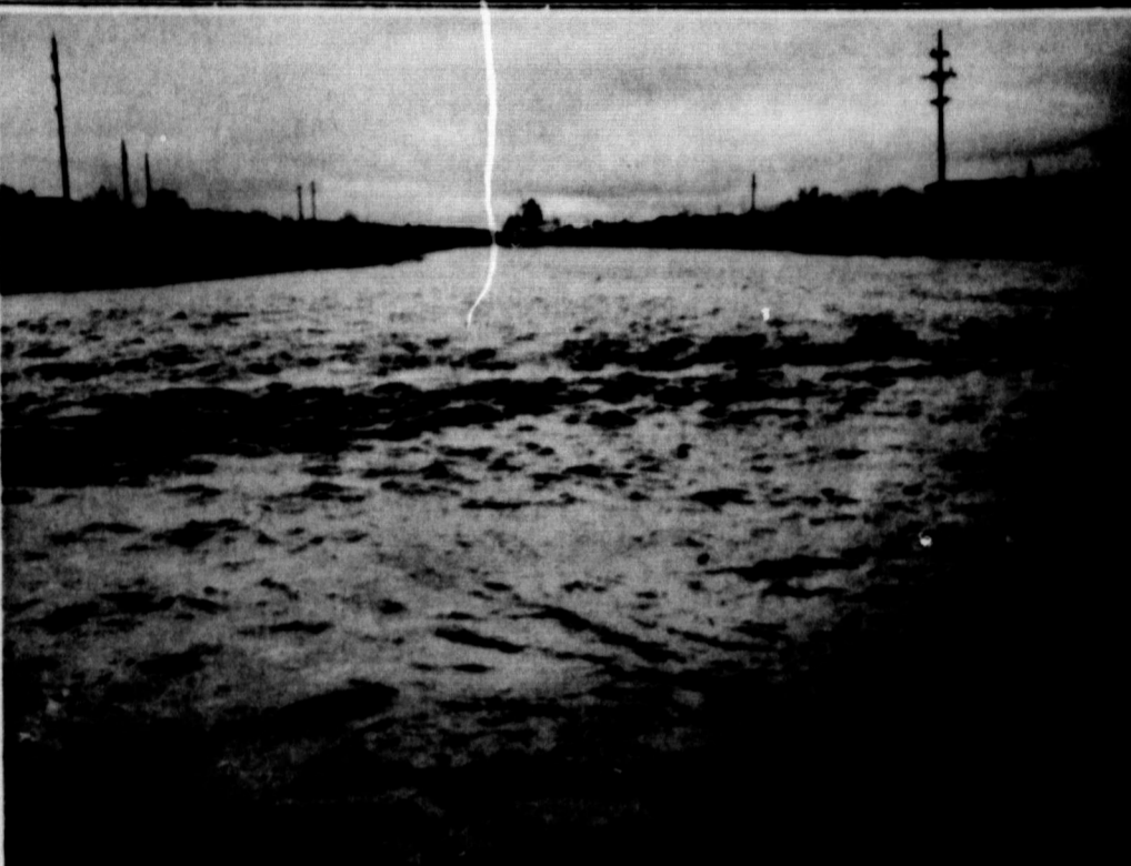
SINCE NOBODY-CAN-REMEMBER WHEN has this sight greeted eyes of Ozonans. It is Johnson Draw tumbling along from bank to bank after last Thursday night's heavy rains here and upstream. The run-off in Johnson through town comes from small draws below the six flood control dams upstream which restrict the draw's flow in case of flooding rains.
