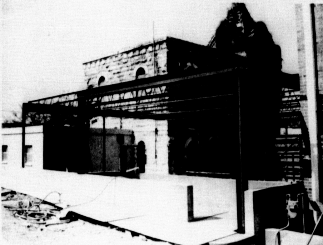
NO MORE INVITING perhaps than the old one but the new Crockett County jail now a-building is certain to be more convenient for authorities and a safer place for incarcerating criminal characters. Steel framework is rising on the new jail project which will form an addition to the present facilities to make it possible for this county to have suitable jail facilities to take care of female and juvenile prisoners. Presently such prisoners must be taken either to Big Lake or Sonora.
