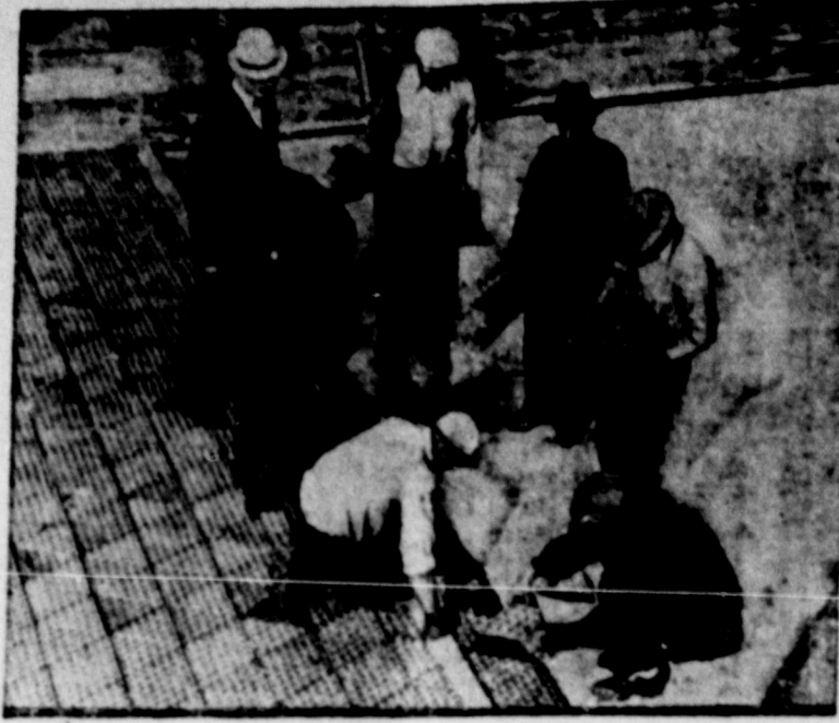
Cast iron paving made its debut in the United States when a thirty-foot strip was laid at the University of Minnesota in Minneapolis for a test to determine its possibilities on a national scale.
