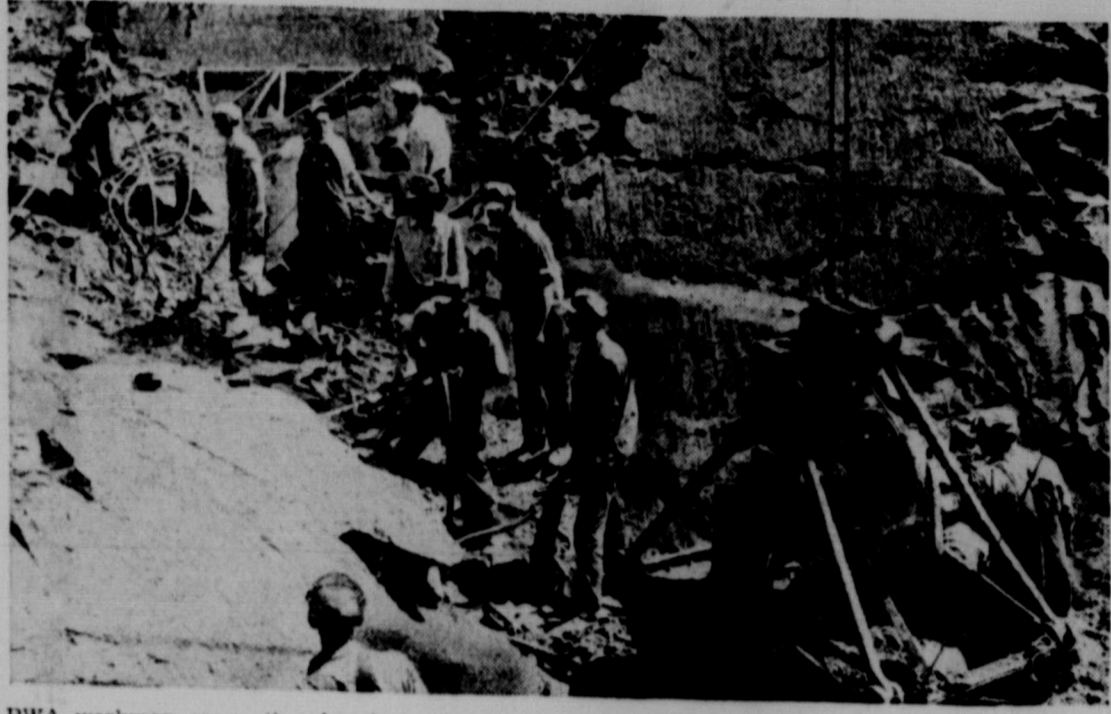
PWA workmen excavating for the spillway structure of the Fort Peck dam, a project in eastern Montana, financed in part by an allotment of $49,881,000, from the Public Works administration. When completed, the Fort Peck project will be the largest earth-fill dam in the world, will control floods of the Missouri river and irrigate thousands of acres of now arid land.
