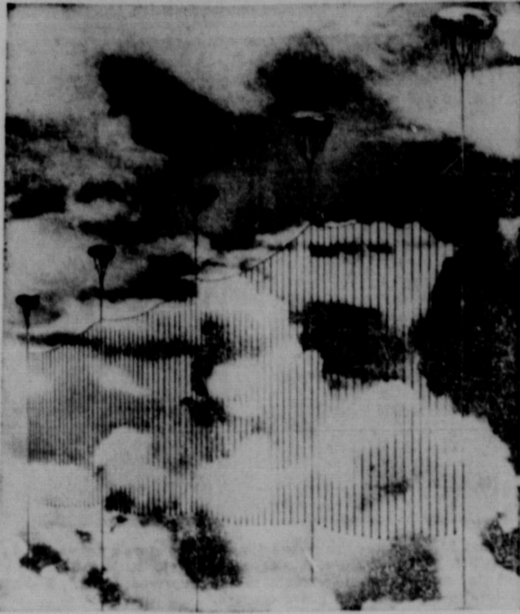
In the next war London may be defended from enemy bombers by great cable nets supported by balloons like that shown here. It is a revival of a plan of 1917 and provides a menace to low-flying planes, forcing them to fly higher, where searchlights, range finders and aircraft guns may be used against them more effectively.
