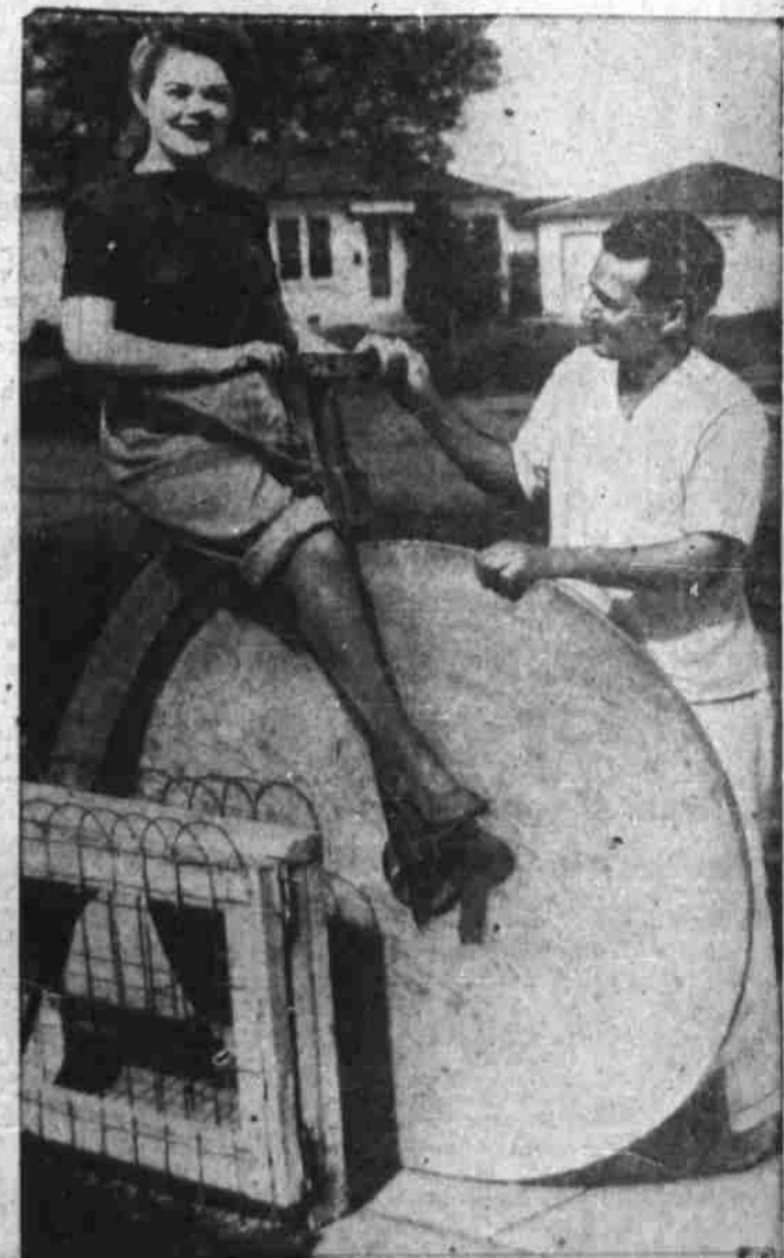
WHO'S WORRIED ABOUT TIRES? —One answer to the rubber and metal shortage is this "wooden wacky" bike, built by Dr. Don Truitt, Long Beach, Calif., cyclist, who shows Lorraine Foreman how to ride it. It's made entirely of wood except for bolts, pedal gear.
