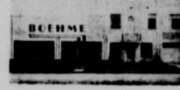
Our New Plant, Built in 1941
