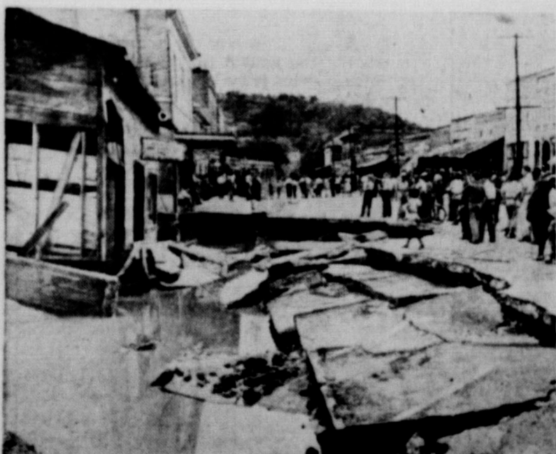
Undermined by flood waters from a swollen tributary of the Alabama river, this section of the Prattville, Ala., main street collapsed, halting traffic through the business district. Floods were caused by heavy rains, and though there was no loss of life, more than 3,000 persons in the southern part of the state were forced to see their homes.
