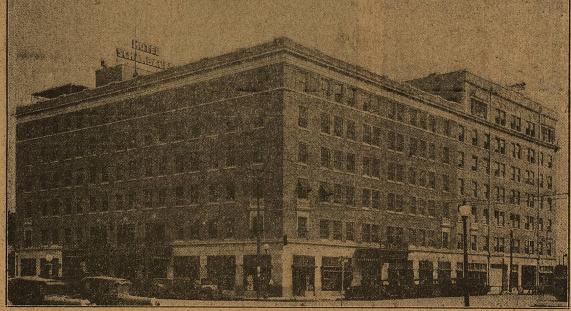
The Scharbauer hotel, built by Clarence Scharbauer and wife and formally opened to the public April 13, 1928. At first a hotel of 150 rooms, after being open for only one year 100 more rooms were added to facilitate handling of the large crowds inevitably in attendance at the building. It was erected by Scharbauer and wife at an estimated cost of $750,000.
