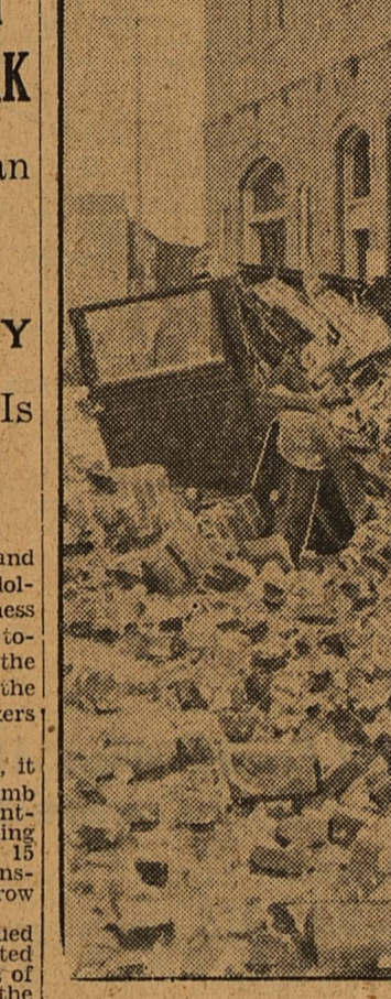
Size of the reconstruction task facing Helena is indicated by this picture, a scene of ruin along one of the capital's main streets, damaged heavily by the recurrent quakes. An automobile parked near the stores is seen after an avalanche of bricks had plunged down on it from business structures in the latest series of shocks that made thousands flee the city.
