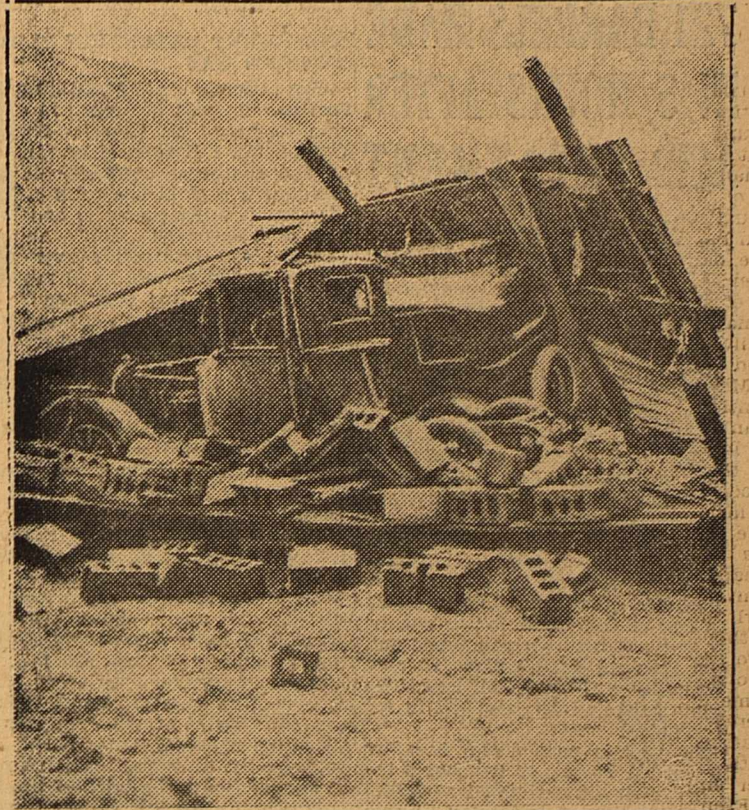
This scene was typical of ones prevailing on hundreds of back lots of the flooded district after the torrents had subsided. Just a shattered heap of lumber and cement blocks now, the structure caved on the two cars when the surging waters raged through the streets of McKee Rocks, Pa.
