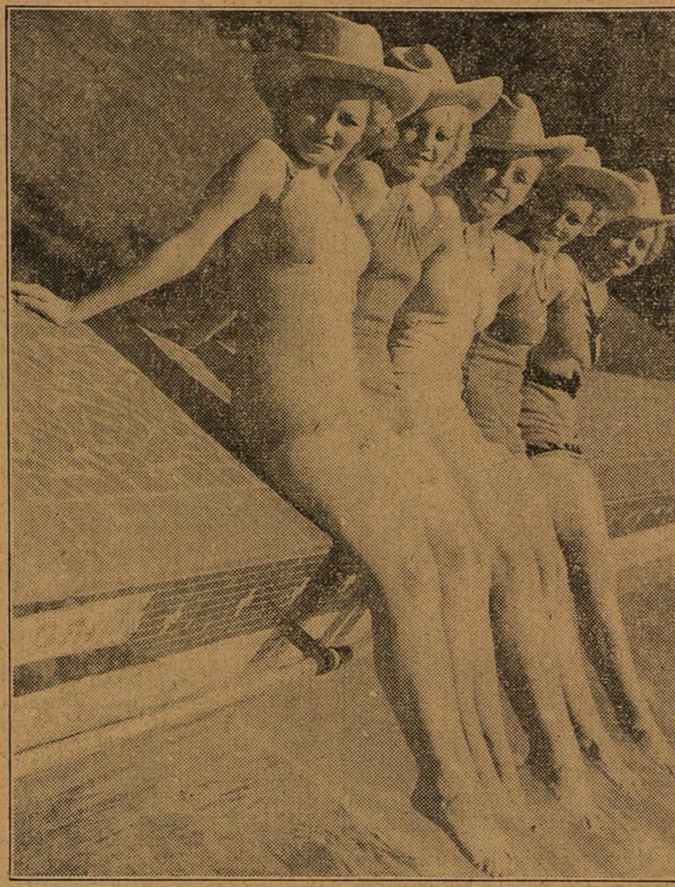
Those Rangerettes of the Texas Centennial Exposition, which will open in Dallas June 6, can't seem to go anywhere without their 10-gallon hats. Here are five of them trying out an already completed Exposition swimming pool behind the $5,000,000 Midway.
