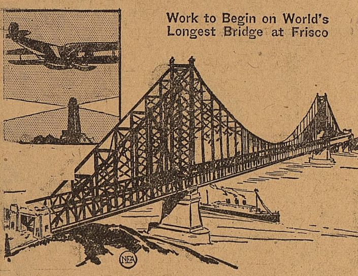
Work to Begin on World's Longest Bridge at Frisco
