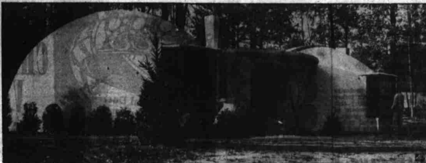
NECESSITY MOTHERS A NEW ONE —To satisfy demands for simple, inexpensive homes in defense production centers, his experimental kloo-type house was built in Fairfax county, Va., workmen spraying concrete mixture onto inflated rubber forms.
