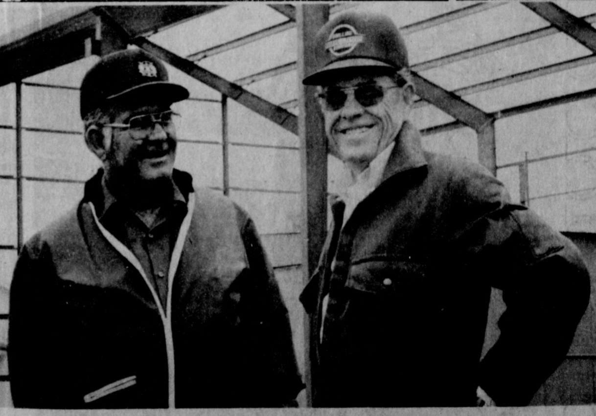
Dick Kilgore on the left, and Roy Bulls on the right stand beside the new framework for the Baker-Taylor building in Spearman. The new addition will enlarge Baker-Taylor's shop to near 23,400 square feet. Kilgore is construction foreman for some of the building projects, and Bulls is a Baker-Taylor employee.
