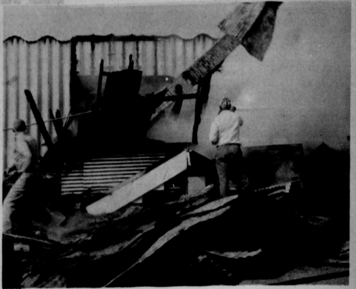
CHIMNEY GOES DOWN— Firemen pushed the chimney of the Morse Oil Co. over as other firemen pour water on the smoldering rubble. The building burned Monday morning.
