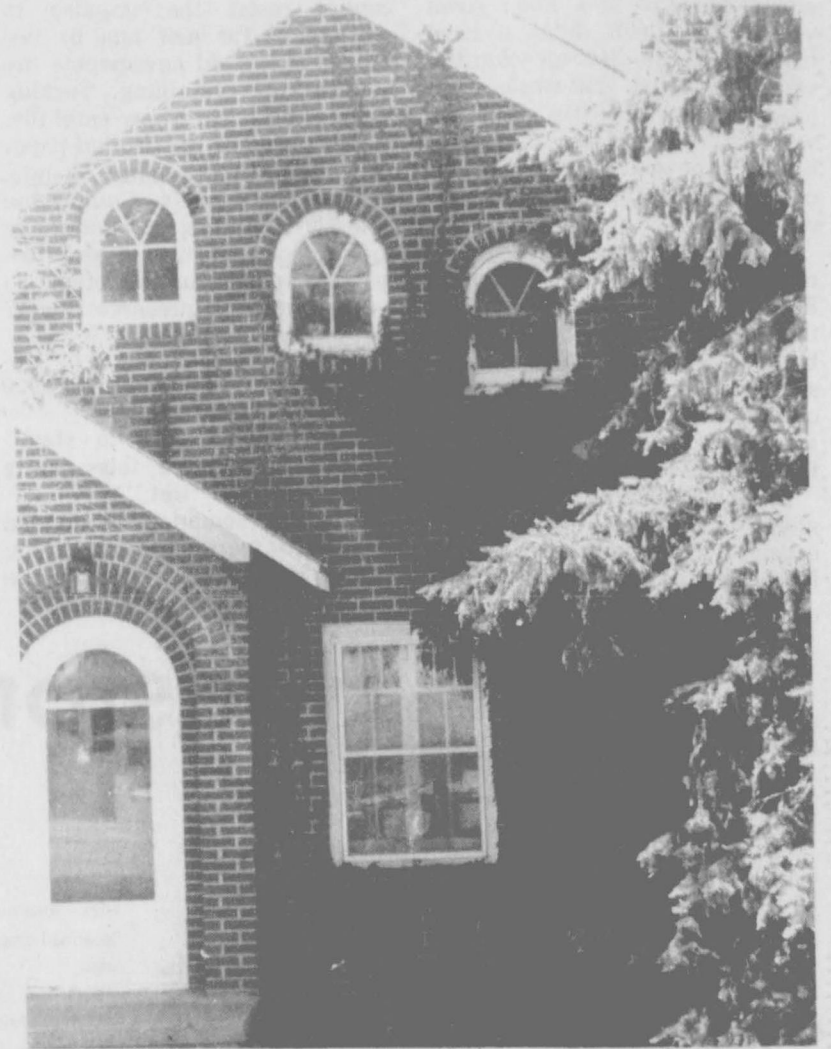
Gruver's second brick house was built in 1929 by the J.H. Gruvers. Located at Broadway and Womble, the elegant home is owned today by family descendants.
