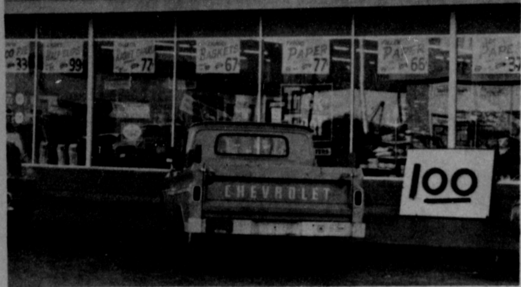
DOLLAR LOST--The wind Sunday afternoon sent prices down about 12 feet at the Spearman T.G.&Y. store. Wind blew the $1.00 off the store sign leaving prices low. No damage was done to the building.
