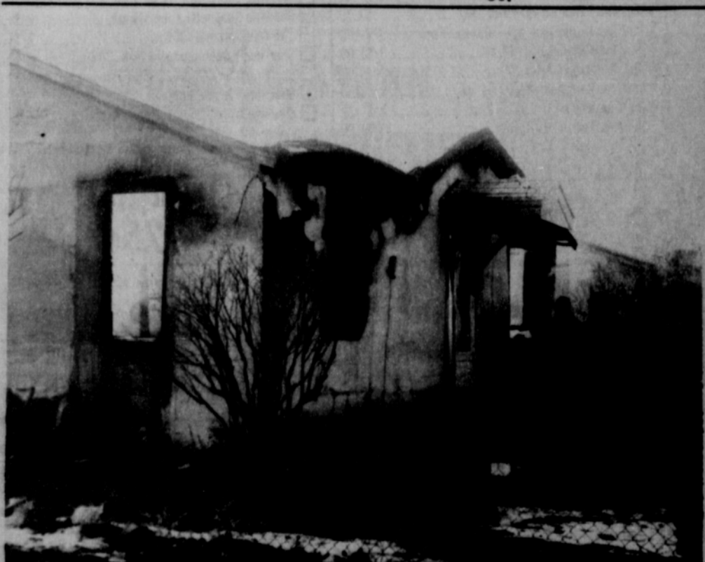
SECOND TIME- Spearman Volunteer Firemen pour water into the smoldering hull of a vacant house on S. Hazelwood. The house burned early Tuesday morning, then had to go back the second time to kill the blaze.
