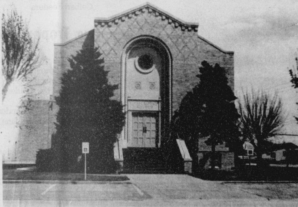
First Baptist Church 123 South Bernice
