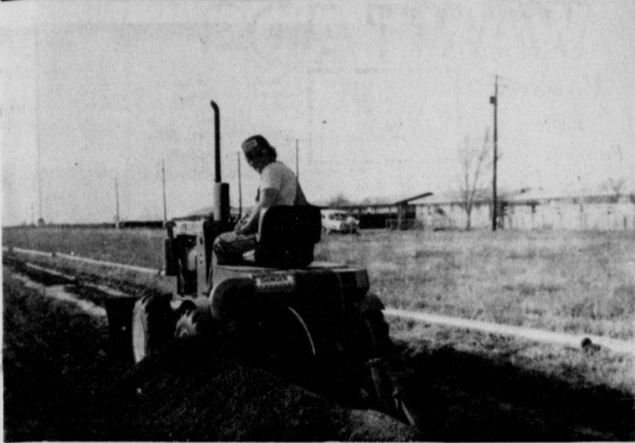
Donnie Carnes of Amarillo and native of Booker is operating this little digger, the latest model Ditch Witch which is, upper photo, opening up the small trench which, lower photo, will be used to carry the new gas line west to the junction of the County road and South Seventh. The project is being done by T.O.K. Company of Amarillo as part of Economic Development Administration projects in Spearman. When completed, this work will have included new line installations as well as improvements to the existing system.
