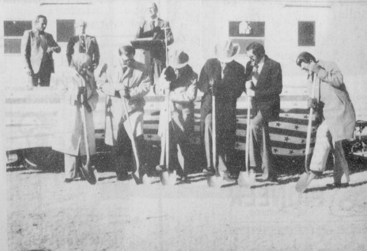
MOMENT OF JOY -- Turf was turned Friday to officially start work on the new extended care center From the left, Mrs. H. N. Shedeck; Mayor Blodgett; Bill Etling, hospital board vice-president; Gruver Mayor J. C. Harris; County Judge R. L. McClellan and Rev. David Nuckels. On the platform from the left, Glenn Harris; Mark Hardin, hospital administrator and Rev. Russell Pogue, MC. Mrs. Shedeck was representing the Home Demonstration Clubs.
