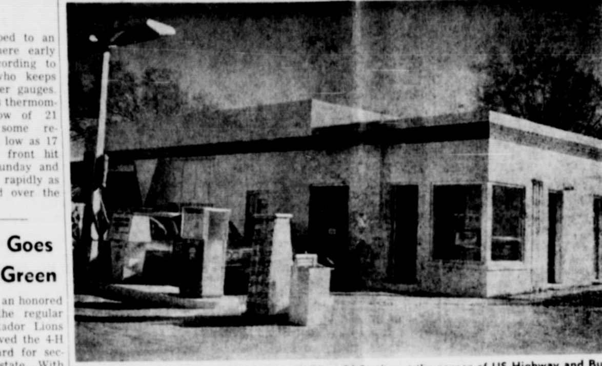
CHANGING SCENE IN MATADOR— Phillips 66 Station at the corner of US Highway and Bundy Street looks different now. The station is now the property of Howard Edmondson, who has recently completed extensive remodeling and improvements. Enclosed wash and grease rooms are at the left of the remodeled old station built by the Phillips Co. more than 30 years ago.
