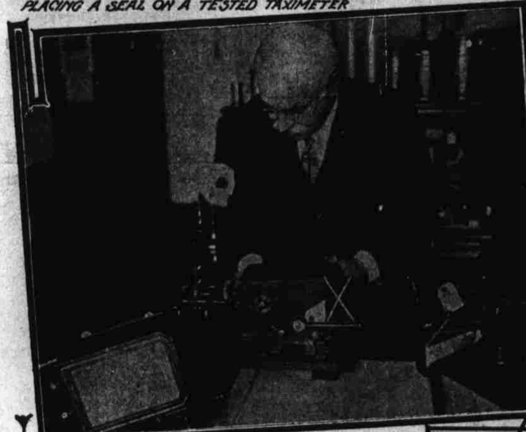
ATTACHING A TAXIMETER TO THE NEW TESTING MACHINE
