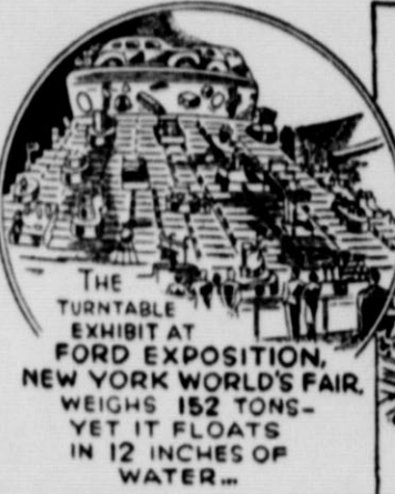
THE TURNTABLE EXHIBIT AT FORD EXPOSITION, NEW YORK WORLD'S FAIR, WEIGHS 152 TONS - YET IT FLOATS IN 12 INCHES OF WATER...
