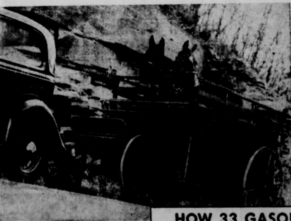
A BORROWED FORD tests 12 competing gasolines on Muldrough Hill, near West Point, Ky., to see which gas can pull the car and 3500-lb. load farthest up hill in high gear.
