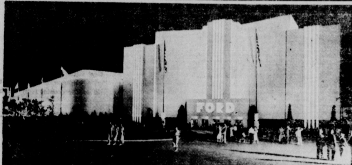
Its solid white walls flooded with many lights, the huge Ford Exposition building at the Texas Centennial in Dallas makes an attractive and imposing structure at night. Parapet lighting adds beauty to the design. The front of the building, which faces Federal Concourse, has rows of Neon tubing which contribute much to the general lighting arrangements.
