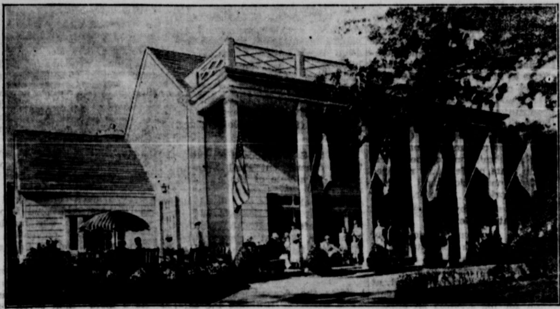
This authentic old Southern Colonial mansion built on the grounds of the Texas Centennial Exposition at Dallas by the Continental Oil Company is for the free use of Exposition visitors seeking a cool haven of rest and relaxation. Air-conditioned, and located just inside the Exposition gates, "Hospitality House" has played host to nearly all comers since the Exposition opened June 6.
