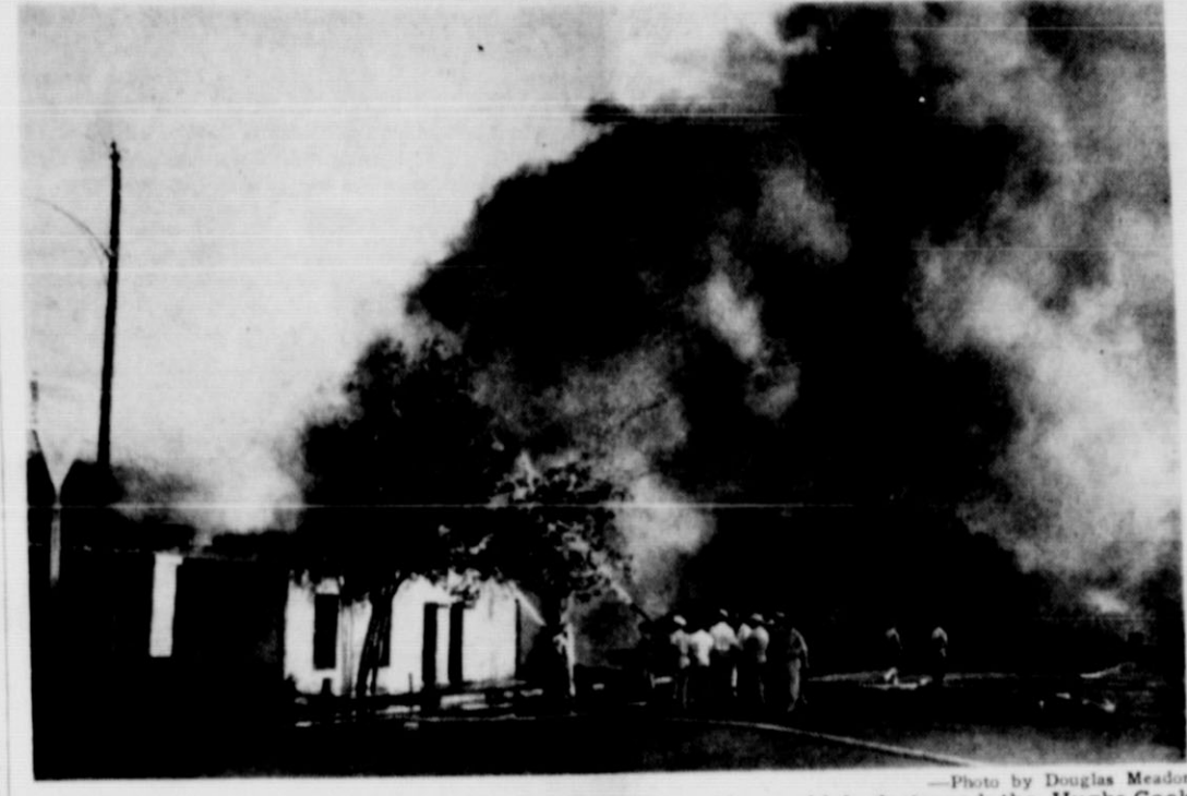
FIREMEN IN FUTILE EFFORT to check the stubborn blaze which destroyed the Hughs-Cook Implement Company, service station, and Conoco wholesale agency office last week, are shown in the above photograph. Billowing black smoke obscured the First Methodist Church as the fire raged beyond control. Loss of the building and contents was estimated between $25,000 and $30,000. The building was a mass of flames before the alarm was sounded. Cause is believed to have been a spark from a grinder which ignited spilled gasoline.
