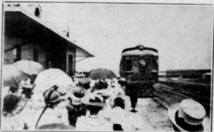
ROARING SPRINGS DEPOT in 1914. Crowd gathered to watch the train come in from Quanah. This is a gasoline-electric motor car, later replaced by a steam train. Note four large umbrellas and women's hats.
