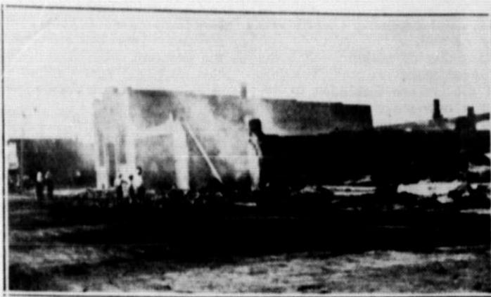
DISASTROUS FIRE , which destroyed most of the business section of Roaring Springs, is depicted in his picture. The blaze occurred in February, 1915.
