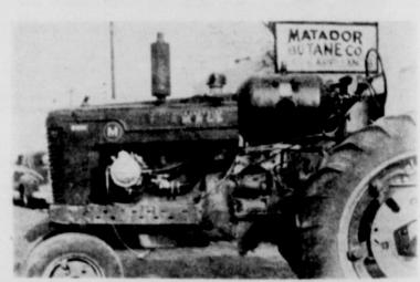
It is easy to equip your tractor to burn Butane Gas. The above photo shows a Farmall tractor with the Butane fuel tank and carburetor in operation. You can earn more profit from farming by saving up to one-half on the cost of fuel.
