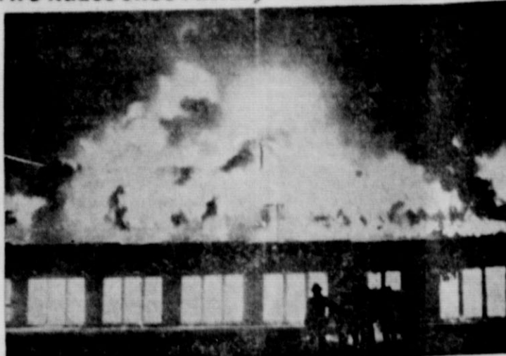
PASADENA, Calif.—Fire causing a loss of one million dollars and throwing 300 persons out of work destroyed the Joyce Shoe factory here. Nine fire companies kept the blaze from spreading to adjoining buildings, and no one was injured.
