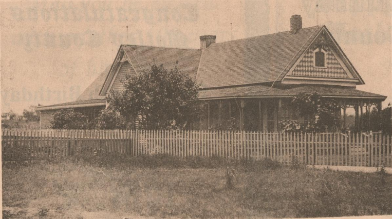
The home of the Walter Waltons, built in 1900. Lumber was hauled from Childress. It was located in the middle of the street, from Steve Burns home. It was moved in 1926 and now is the home of R.C. Giesecke.
