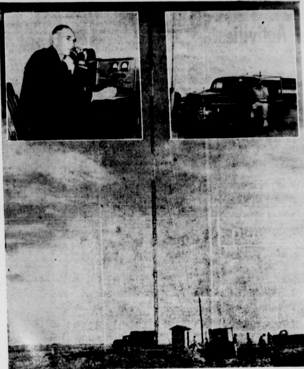
WTU CO.'S NEW TWO-WAY RADIO SYSTEM.—Station KGHQ calling Car J-3, calling Car J-3. That's the call when Carl Hudson, upper left, WTU Co. local manager, Childress, Texas, contacts Bob Adams, WTU Co. Serviceman to give emergency instructions over the new short wave radio system, which went into operation last Friday. Pictured center is the 194.8 ft. antenna of the 250 watt central station located in Southwest Childress. WTU Co. now has seven vehicles operating in the Childress district which are equipped with mobile two-way radios.
